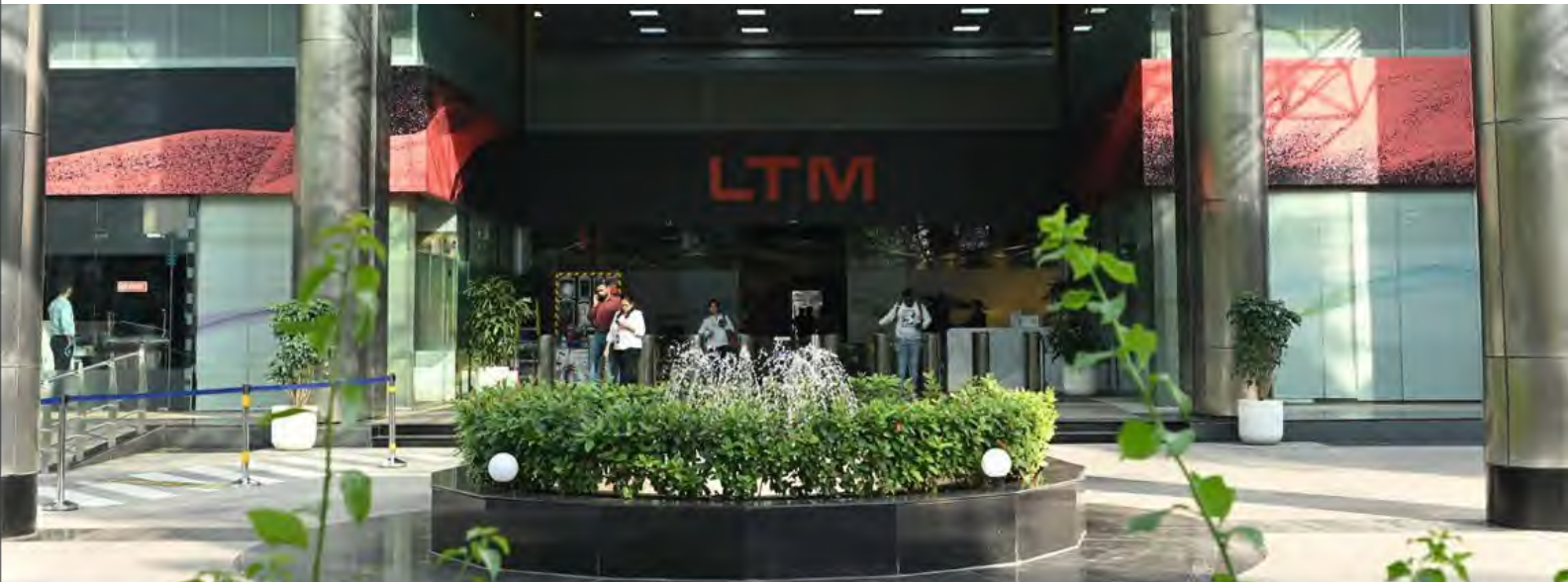
LTM Headquarters, Powai, Mumbai
